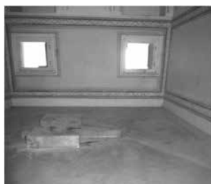
Toilet with Ventilation - Nahagarah fort
