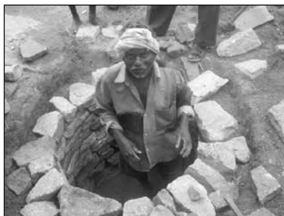
Figure 12 : Toilet Pit constructed using stone
