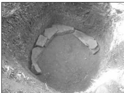
Figure 12 : Toilet Pit constructed using stone
