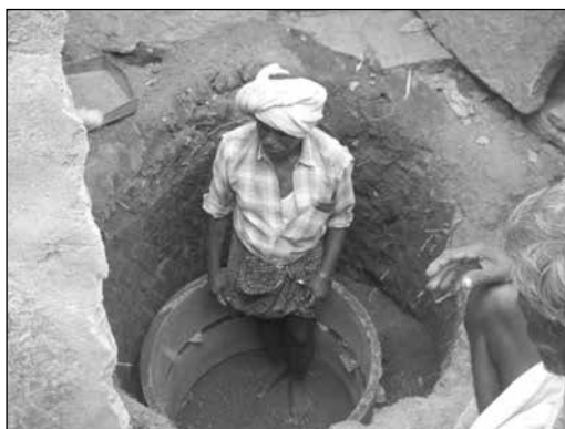
Figure 14 : Toilet Pit Construction using rings
