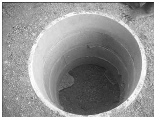
Figure 14 : Toilet Pit Construction using rings
