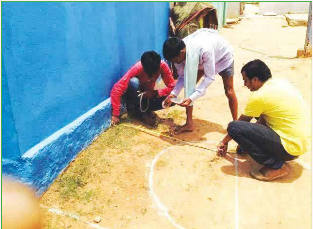
Photograph 7: Masonry training on Toilet Construction at Aralere village.
